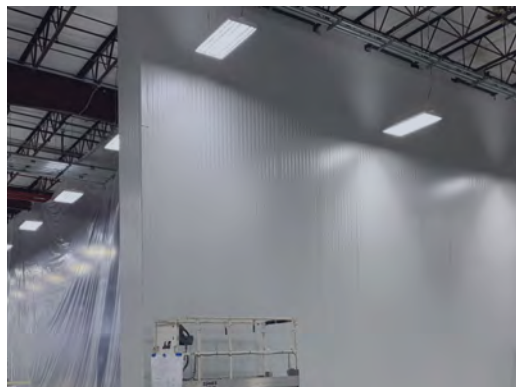
INTERIOR FIT UP
